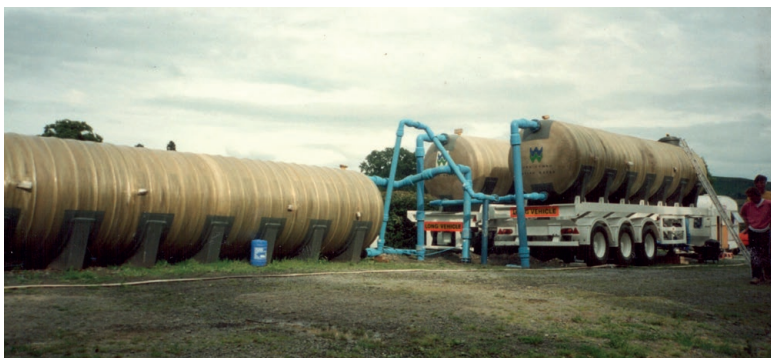
2 x 32m 3 skid mounted emergency water 'standby' tanks – Dwr Cymru/ Welsh Water deployed at the Royal Welsh Show, Builth Wells.
