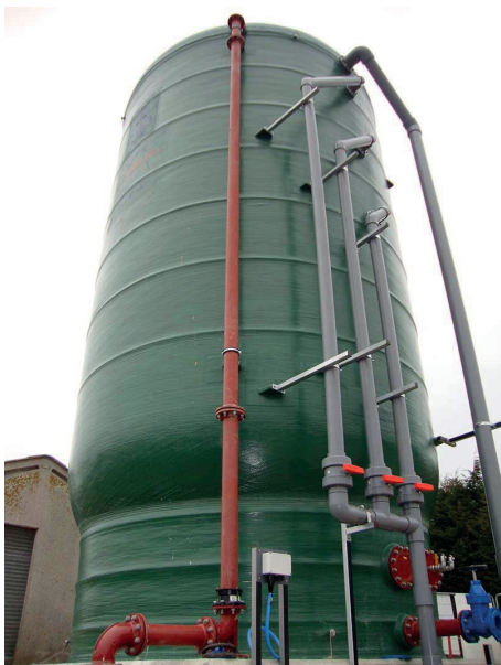
100m 3 sludge settlement tank with liquor decanting valves – one of over 300 in service with South West Water some now 30 years old.
